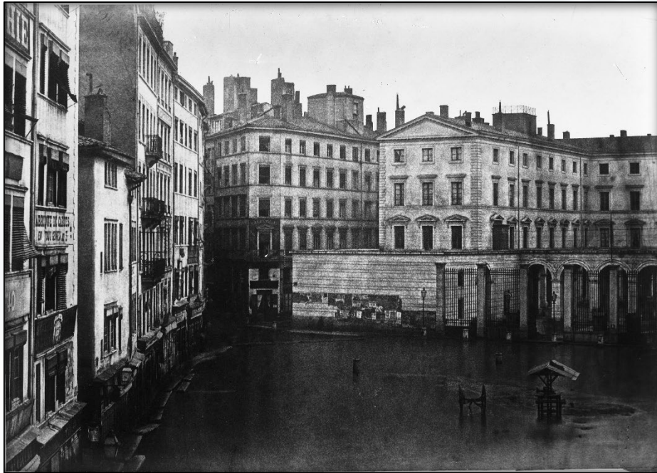
Figure 10 Well of the Place de la Préfecture (des Jacobins) (1856, photo taken during Lyon's river flood)
